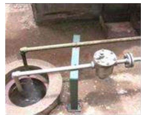
倒筒式祛水器排水洩漏
