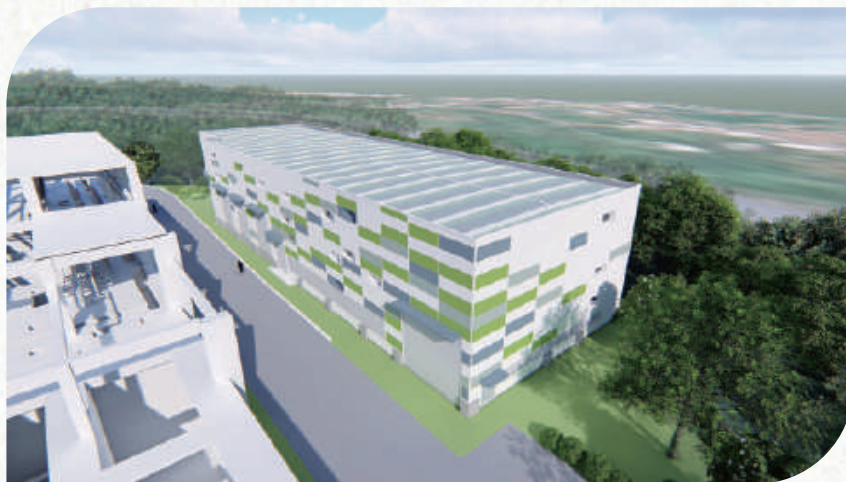
Image of the brine room of sewage treatment plant in Tongluo Park
